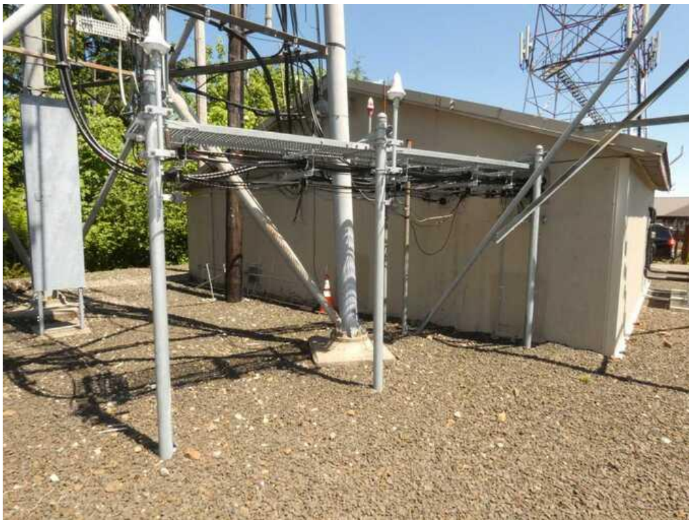
BUSH MTN Cable Ice Bridge
