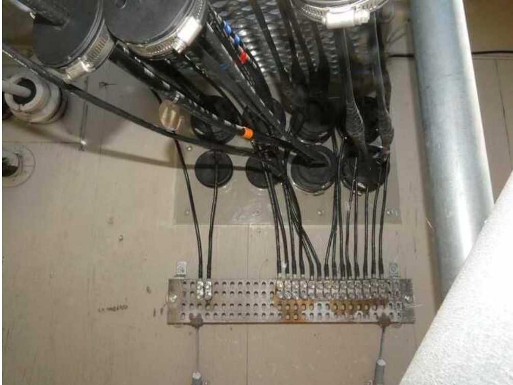
BUSH MTN Exterior Entry Port
